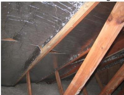
Attic showing reflective bubble wrap and cellulose insulation
