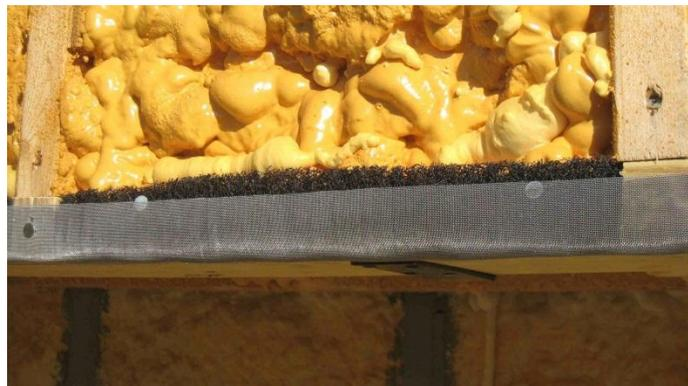
Closed cell foam with Aluminium Mesh
